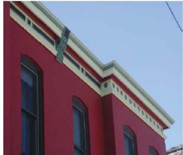
The building front correctly contains a parapet with cornice.
