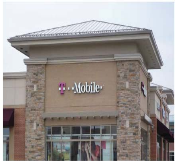
This pitched roof has overhanging eaves.
