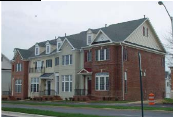
The building properly offsets wall planes.
