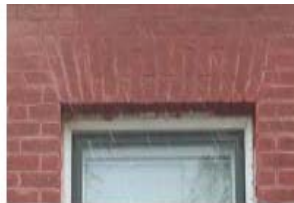
A jack arch above a window opening.
