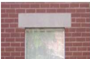
A stone lintel above a window opening.
