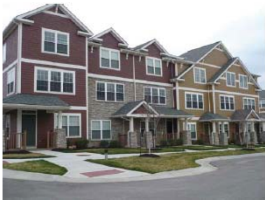
The apartment building limits its length to less than 200 feet.
