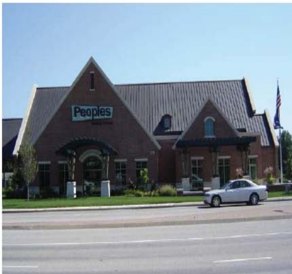
This pitched roof modulates.
