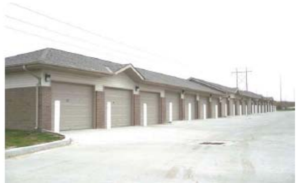
This garage building is over 120 feet long.
