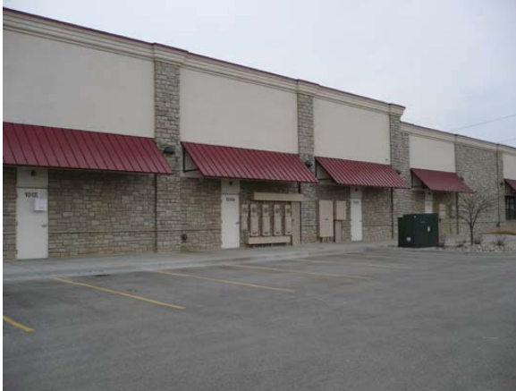
This parapet does not modulate.
