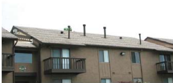
This continuous pitched roof extends more than 50' and does not contain any roof elements.
