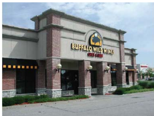
This customer entrance correctly contains columns, display windows, raised parapet, and recesses.
