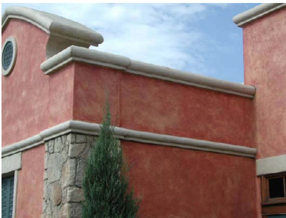
This parapet and cornice returns back into a pitched roof.
