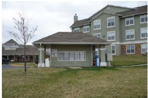
The accessory structure's details and materials are both compatible and consistent with the primary structure.
