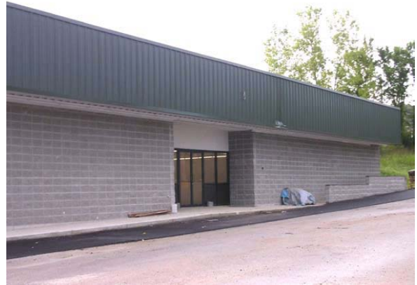
The street-facing facade on this flat-roofed building does not have a cornice.
