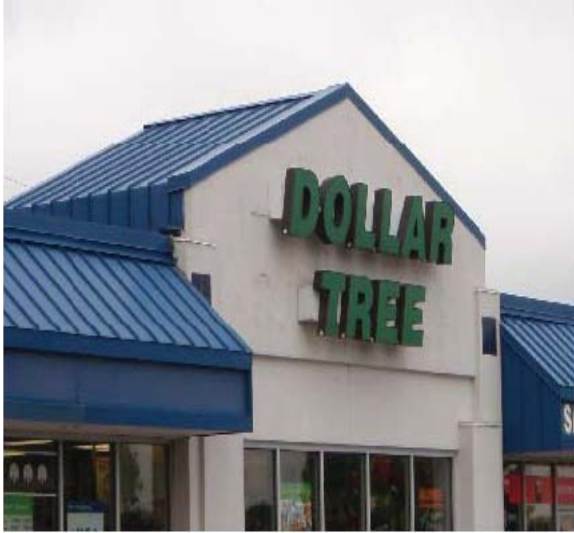
This pitched roof lacks any overhanging eaves.
