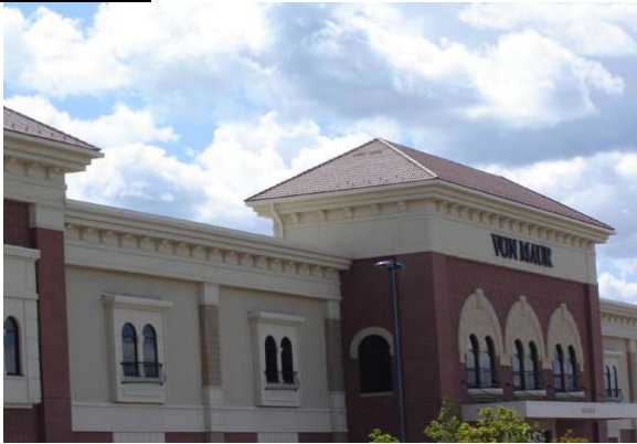
The cornice returns at least 8 feet.
